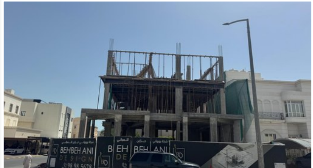
EXTERNAL FRAME PROGRESS
