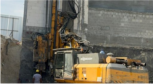
SHORING EQUIPMENT SETUP
