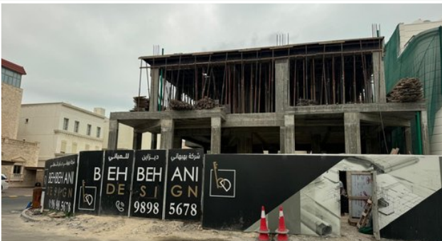
FRONT ELEVATION WORKS
