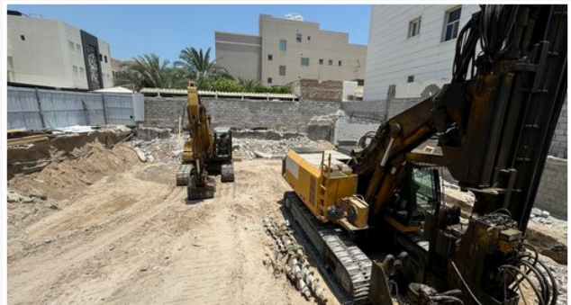
EXCAVATION AND DRILLING
