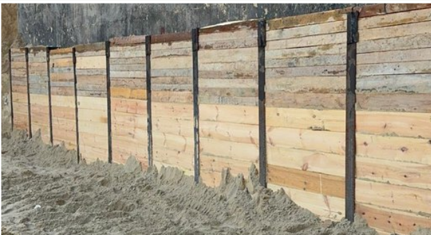
RETAINING BOARDS
