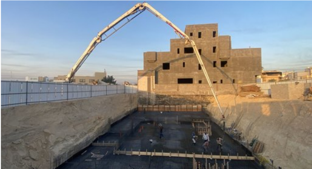
CONCRETE CASTING ACCESS
