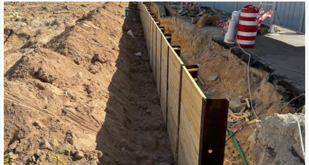
TIMBER LAGGING WORKS
