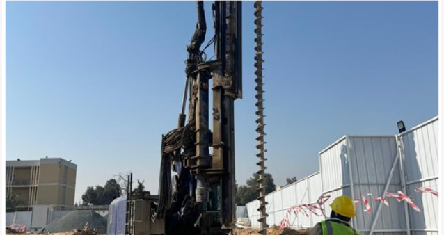
AUGER DRILLING WORKS
