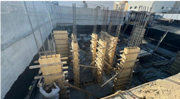
COLUMN FORMWORK
