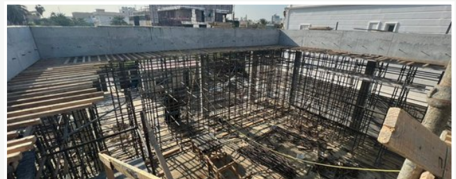
REINFORCED BASEMENT FRAME
