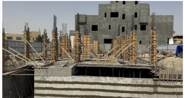
FORMWORK AND FRAME WORKS
