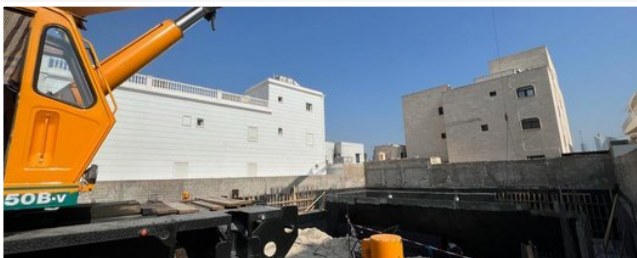
CRANE ASSISTED WORKS
