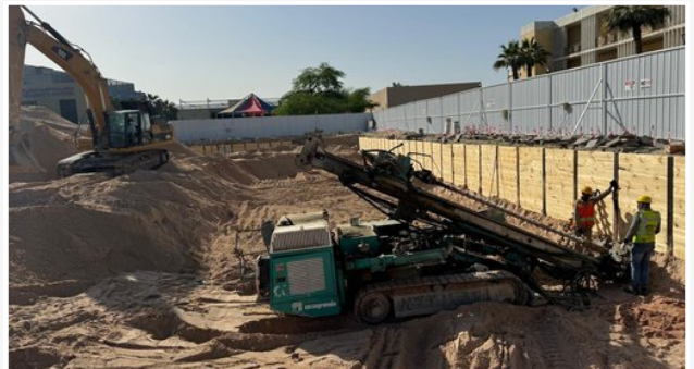
DRILLING AND EXCAVATION
