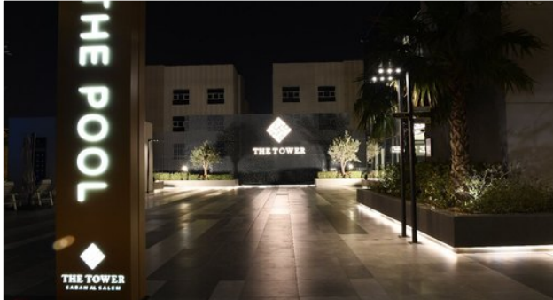
NIGHT ENTRANCE LIGHTING
