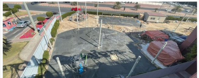
CONCRETE BASE AND POLES
